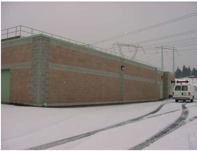
EXTERIOR OF RESERVOIR
