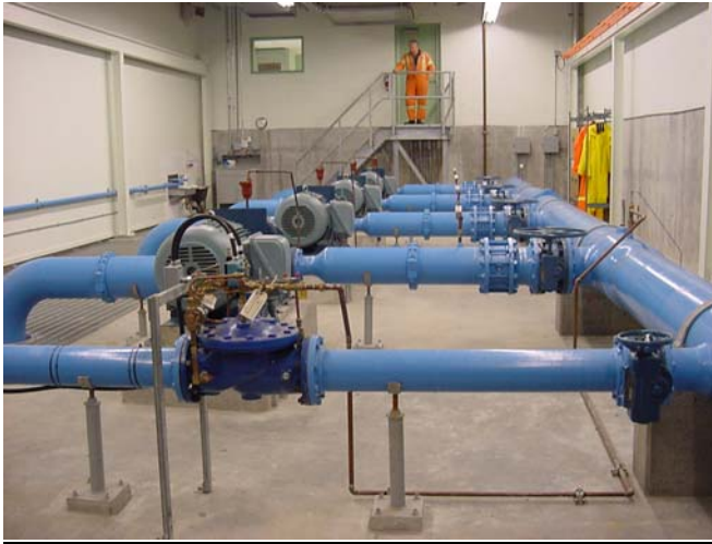
INTERIOR OF RESERVOIR
