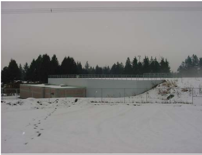
EXTERIOR OF RESERVOIR
