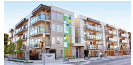
The Serenade high-density residential building project by WestStone Properties in Downtown Langley included an underground airspace parcel for additional tenant parking
